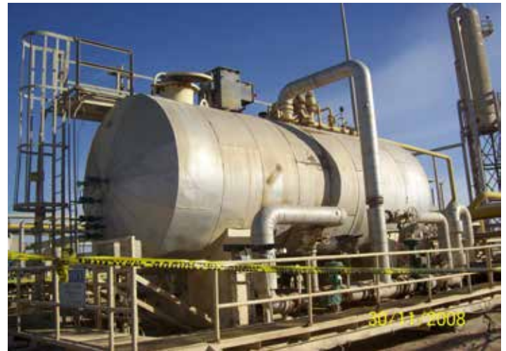
Belzona 5892 used to line a desalter
