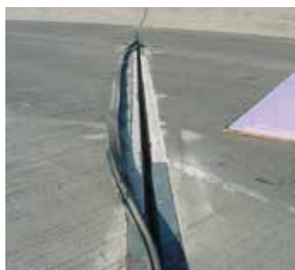
Damaged joint
