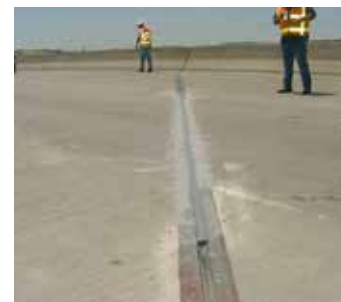
Refurbished joint
